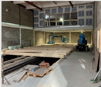
Thompson’s new operation is currently under construction
